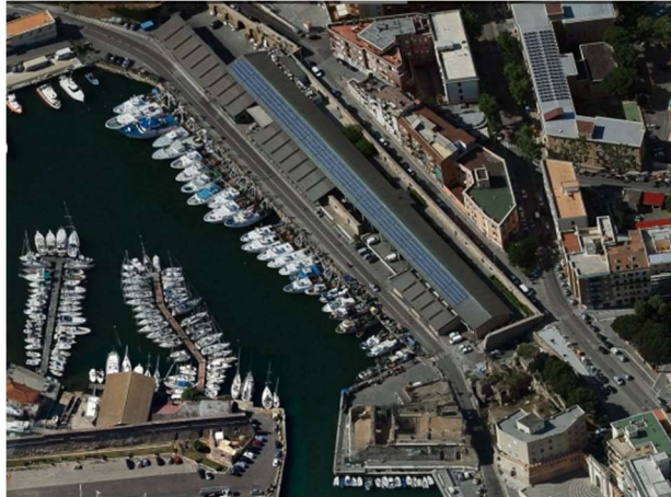
Figure 18 PV 1 PV system on the Darsena Romana
