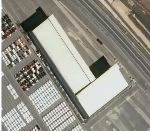
Figure 22 rooftop of the factory Grande Meccanica.
