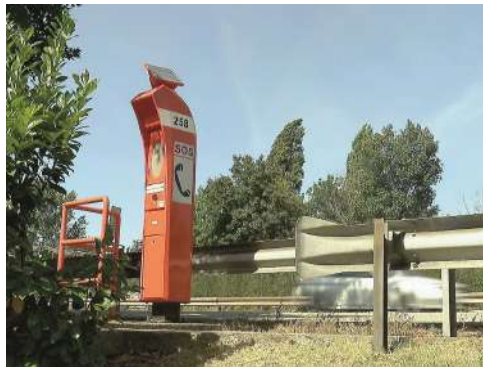
Figure 3.6: Monocrystalline Silicon cell used in an SOS post in Portuguese highways.
