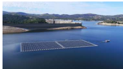
Fig. 1. Floating System in Alto Rabagão dam reservoir, Montalegre, Portugal
