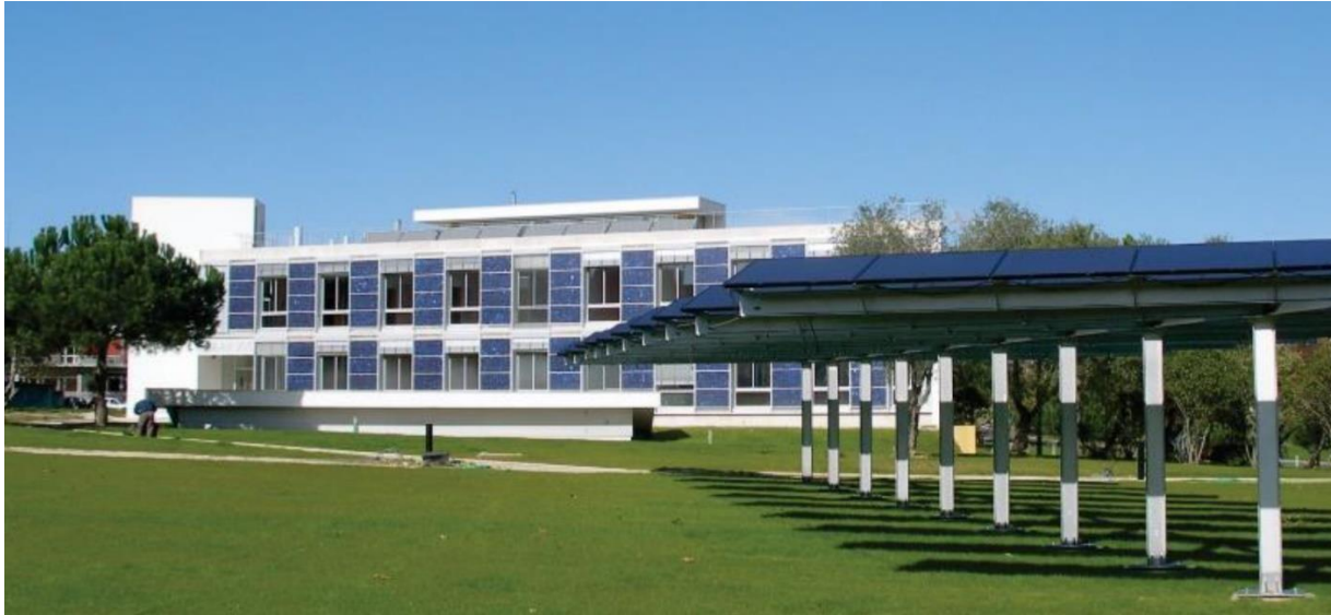
Figure 1 South façade of Solar XXI building and a parking lot located at LNEG campus [23].
