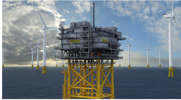
Figure 2.8: Offshore Substation, from [32].
