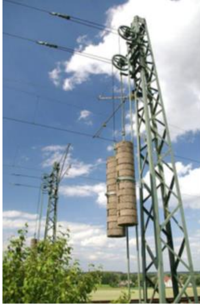
Figure 2.3: Representation of a weights line tensioning system
