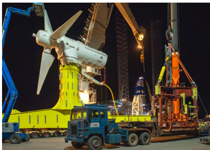
Figure 4: Construction of the MeyGen tidal turbine (SIMEC Atlantis Energy, 2021)
