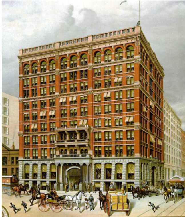
Figure 2.1: Home Insurance Building, Chicago
