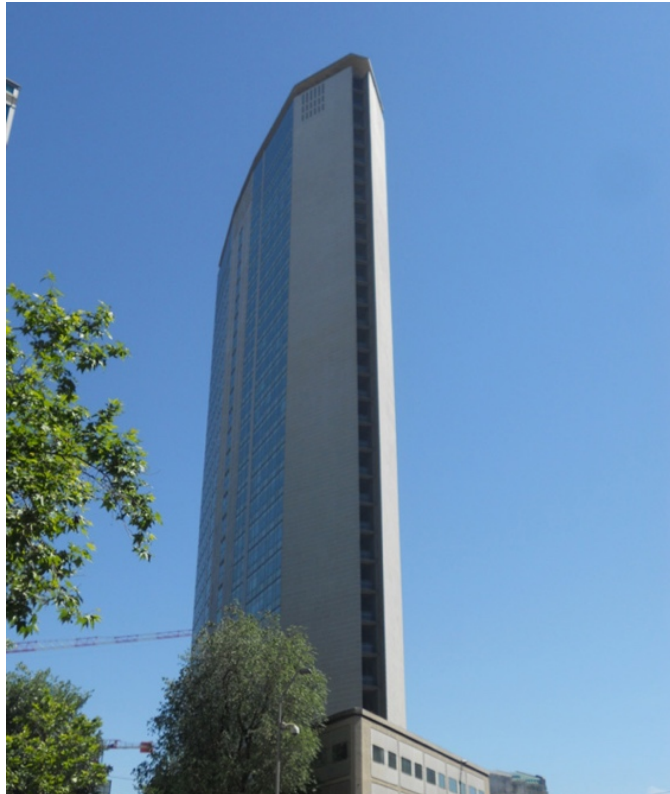
Figure 2.11: Pirelli Building, Milan
