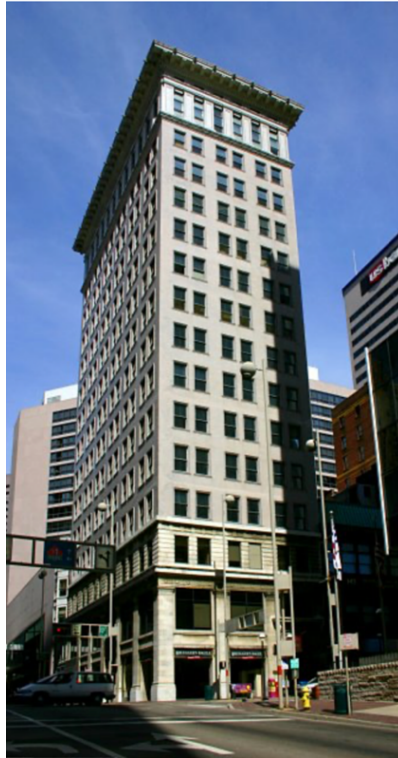
Figure 2.3: Ingalls Building, Cincinnati
