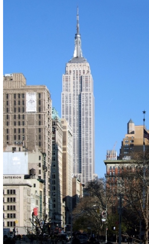
Figure 2.10: Empire State Building, New York City
