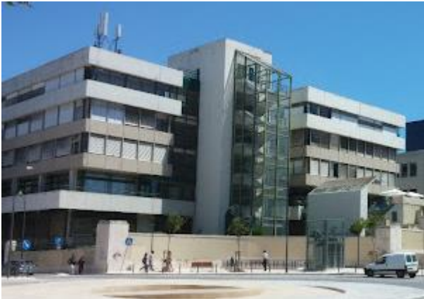
Figure 6 - Side view of the Civil building
