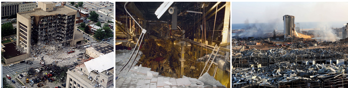
Figure 2.2: Examples of the aftermath of different blast scenarios. First picture from the left, is relative to USA Oklahoma City truck bombing (blast close to surface) [21]. The second image is relative to the USA World Trade Center (underground blast) bombing [22], and the last one, concerning the recent Beirut explosion (blast close to surface) [23].
