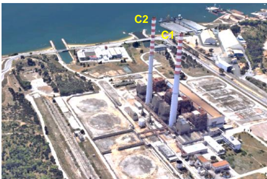
Figure 1.1: Thermo-electrical plant view (Google Earth)
