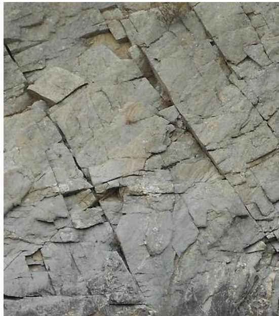
Figure 2.1 Example of joints, source – WhatTheRocksTellUs.com
