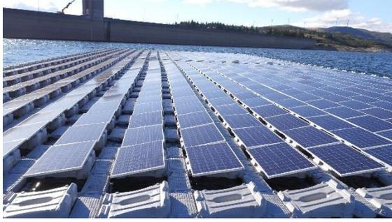
Figure 2 – Floating photovoltaic solar power plant in Alto do Rabação reservoir
