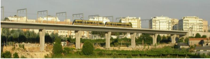
Figure 2.3 - Maia Norte Viaduct [8], [9]
