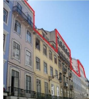
Figure 2.1 – Irregularities in the *pombalino* block due to the increasing number of storeys
