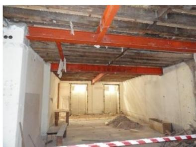
Figure 2.3 – Frontal walls substituted by steel beams [4]
