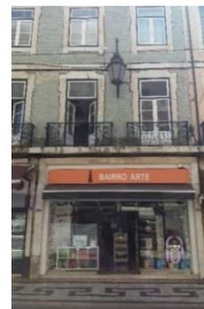
Figure 2.2 – Interruption of piers on the ground floor
