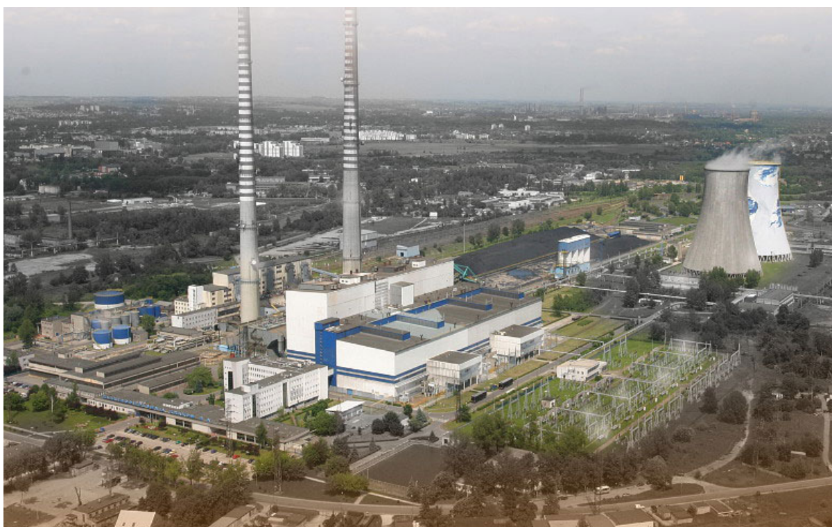
Figure 3.1: EDF CHP plant, Poland, Krakow [9].
