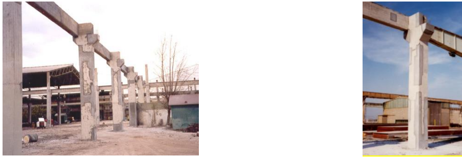
Figure 4: Replacement of concrete with shotcrete on the faces of the columns
