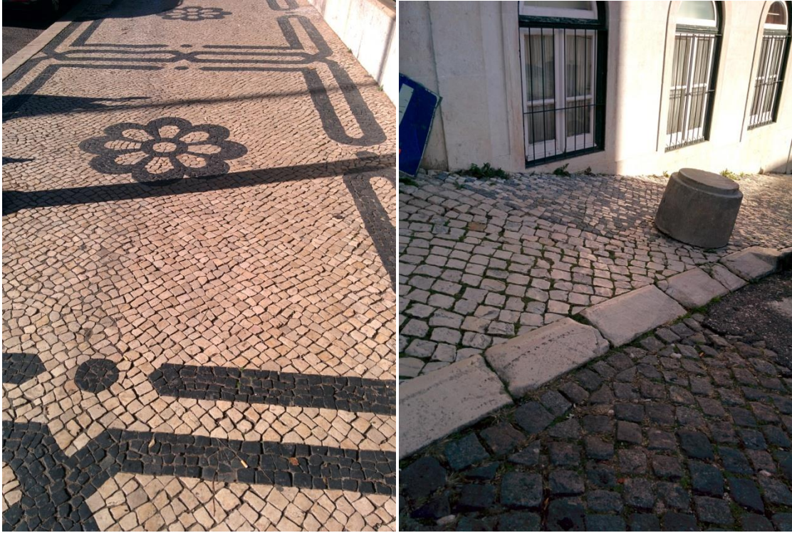
Figure 48- Pavement in very good condition & Slippery pavement and anti-slippery cobblestones
