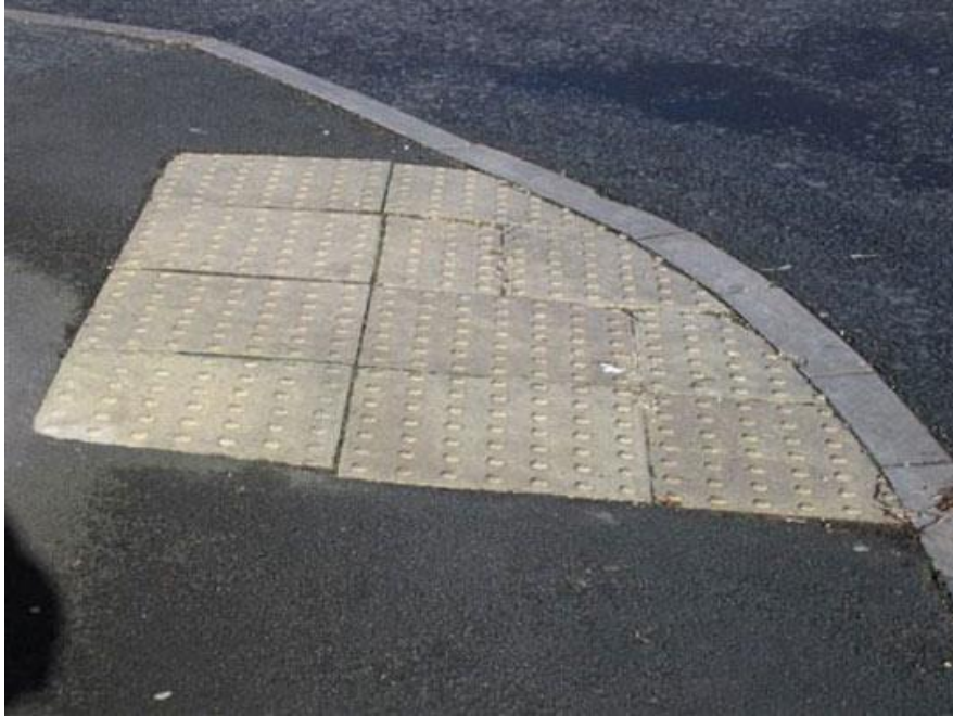
Figure 50-Example of curb drop and tactile aid
