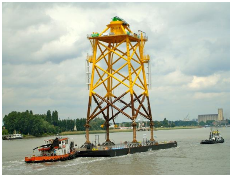
Figure 8- Transportation of the jacket structure [45][4]
