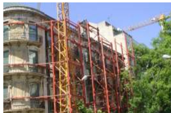
Figure 1 – Temporary steel structure
