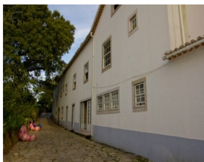
Figura 30 – Fachada – ASH (ASH, 2014)
