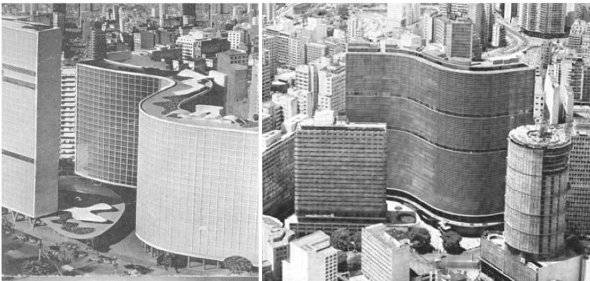
Figure 3 Changes to the Original Project. From left to right: Model of the original design. Source: L'architecture d'aujourd'hui Magazine, 1952 p.42. Aerial photography of COPAN. Source: www.copansp.com.br
