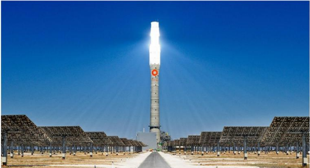
Figure 11. Solar tower with molten salt heat storage near Seville, Spain [25]
