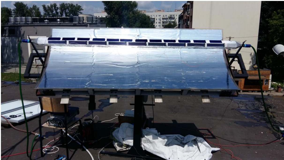
Figure 19. Fully assembled CPVT installation
