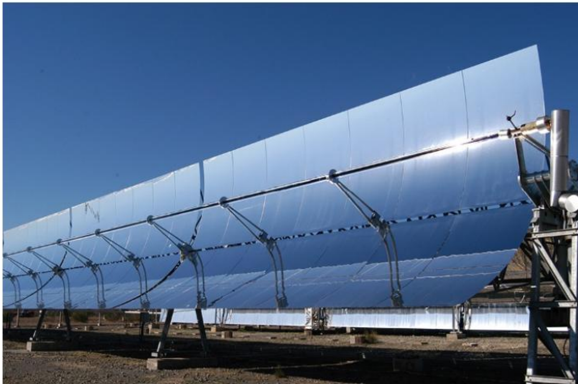
Figure 9. Parabolic trough collector at Solar Platform of Almeria in Tabernas Spain [25]
