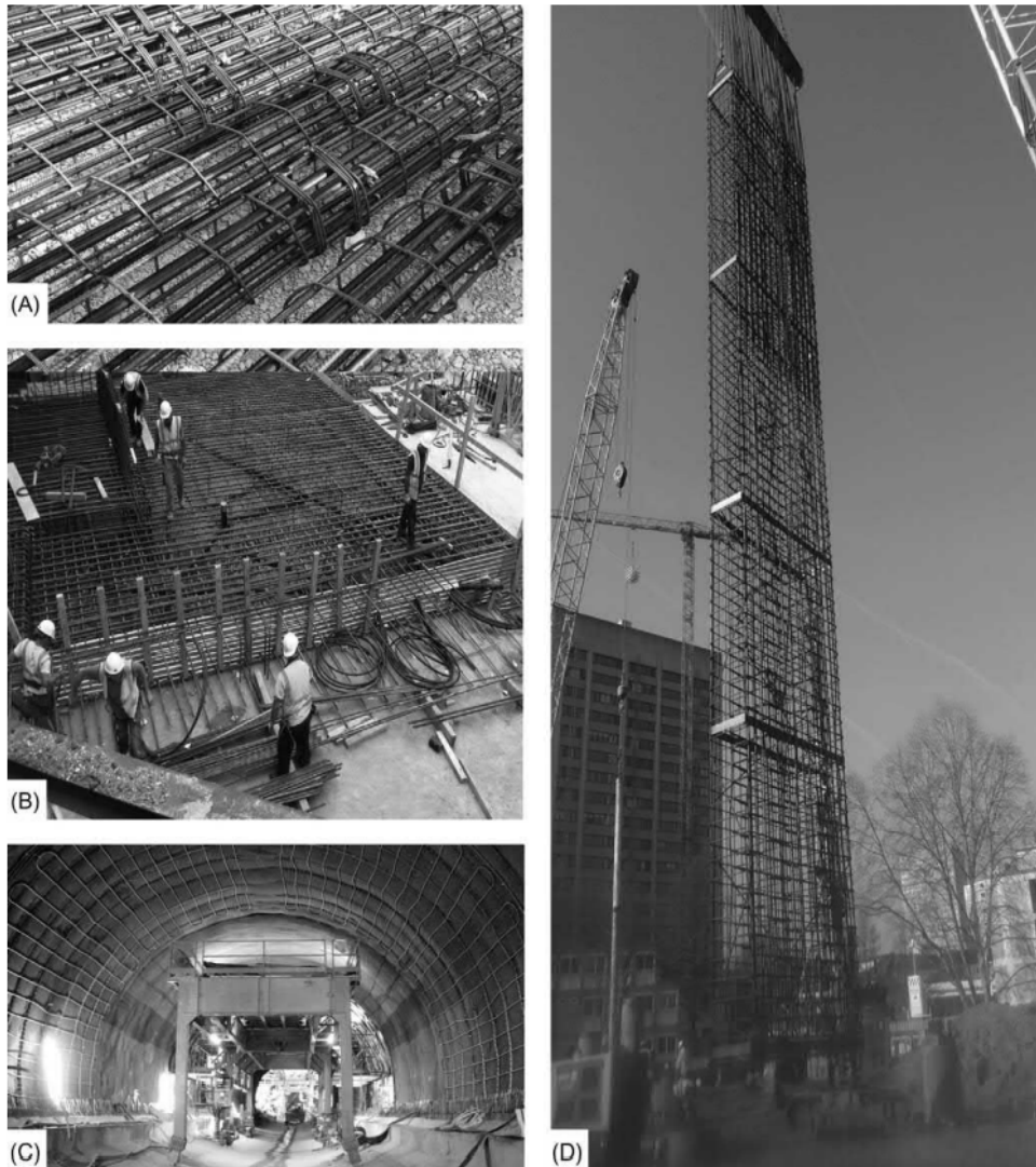
Figure 2.4: Examples of heat exchanger pipes in a) energy piles, b) energy slabs, c) energy tunnels and d) energy walls, (Laloui and Rotta Loria, 2020).
