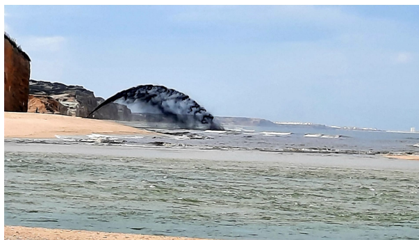
Figure 1.1: Dredging in Foz do Arelho, Portugal (08/2021)
