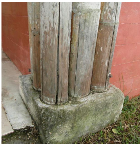
Figure 14- Boron treated bamboo exposed to rain and sun for approximately 10 years showing signs of fungal damage, splitting and bleaching (Kaminski et al., 2016).
