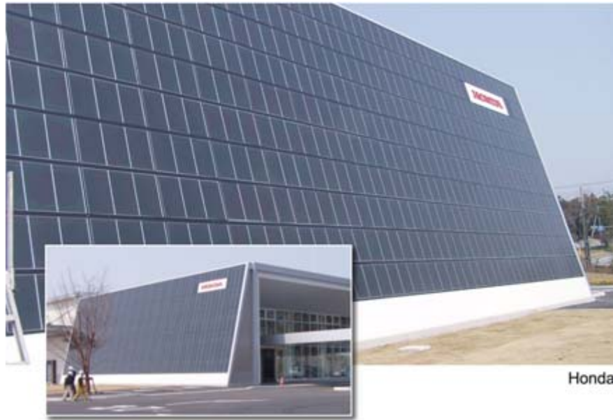
Figure 3.3: Honda Soltec building in Japan, with its thin-film CIGS wall [46]
