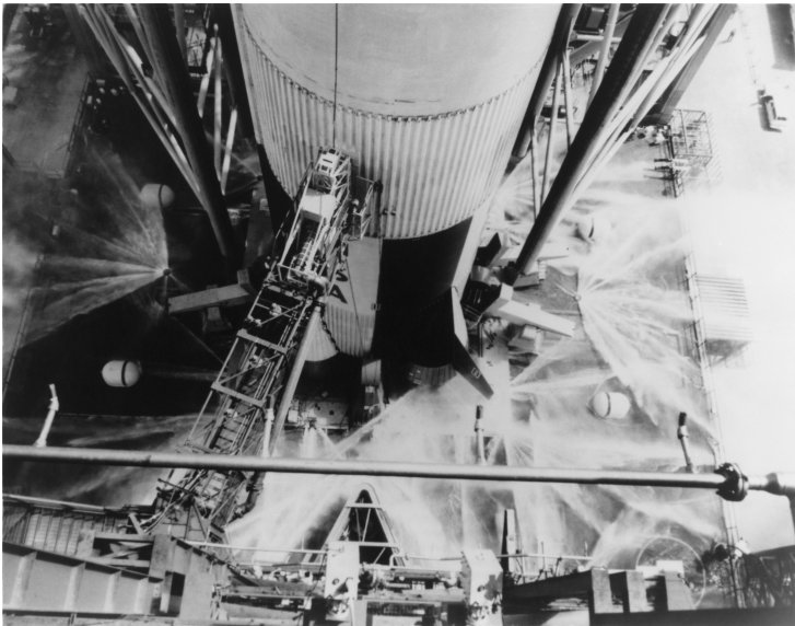
Figure 1.1: Saturn V water suppression system captured during a test. [2]
