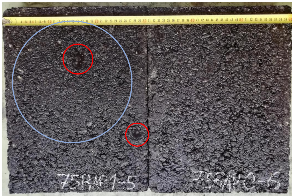
Figure 4.13: Surface texture comparison between 75% RAP (2 nd phase) (left) and 75% RAP (right)
