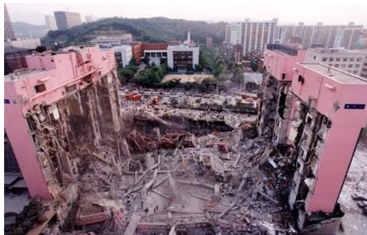
Figura 2.7 Destroços do Sampoong Department Store [Google]
