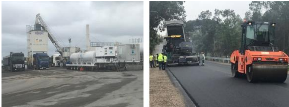
Figure 2-5 Production (left) and application of a bituminous mixture (right)
