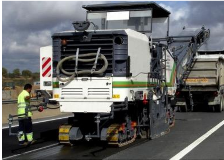
Figure 2-6: Milling of a flexible pavement
