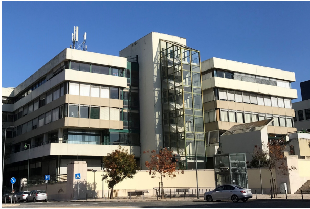
Figure 1: Photograph of Pavilhão de Civil's facade from a southwest perspective.
