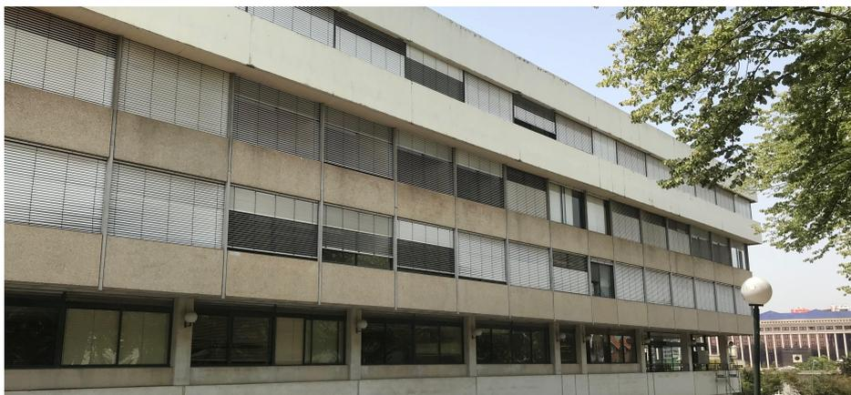
Figure 1.3: Easterly facade of Pavilhão de Civil with the recently installed exterior blinds visible in the 1<sup>st</sup>, 2<sup>nd</sup> and 3<sup>rd</sup> floor. Also visible are the different configurations for the blinds, with slat angle adjustment.
