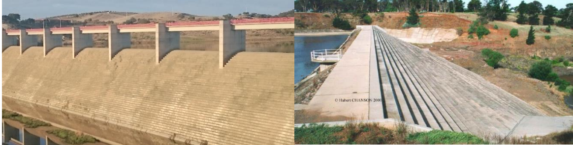
Figure 1 Stepped overflow spillways: (a) Pedrógão dam [5]; (b) Melton dam in Australia [6]
