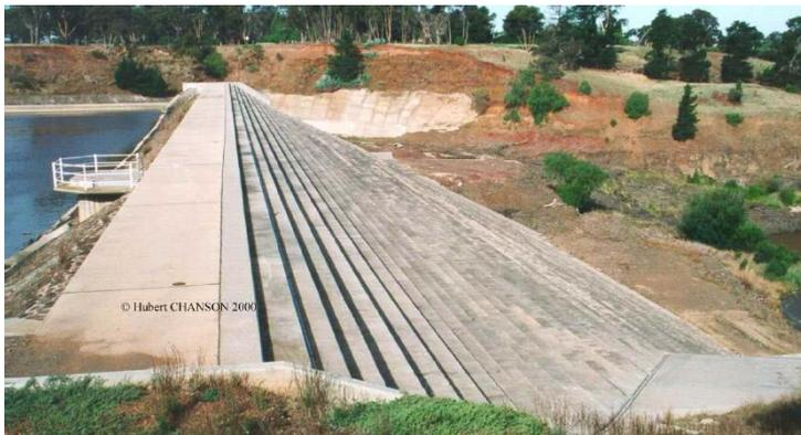
Figure 2-1 Stepped overflow spillway, Melton dam in Australia [4]
