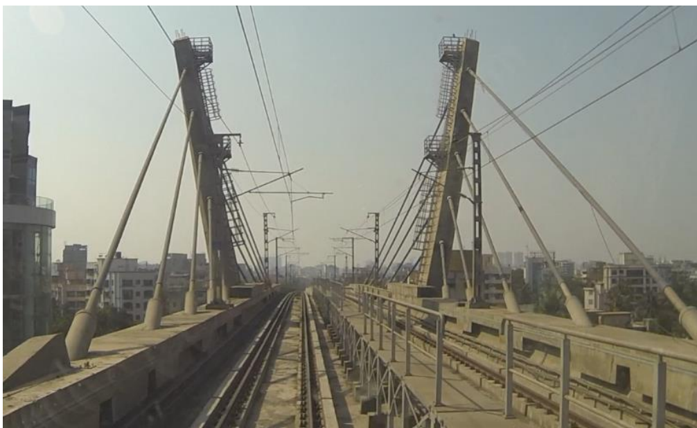
Figure 4.2 - Another Metallic Bridge in the same Mumbai line (extracted from [MMOP14]).
