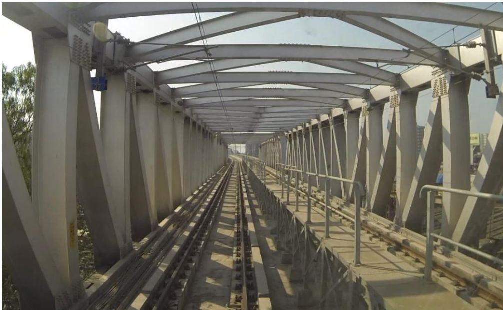
Figure 4.1 - Metallic Bridge in Study, Mumbai Line 1 (extracted from [MMOP14]).
