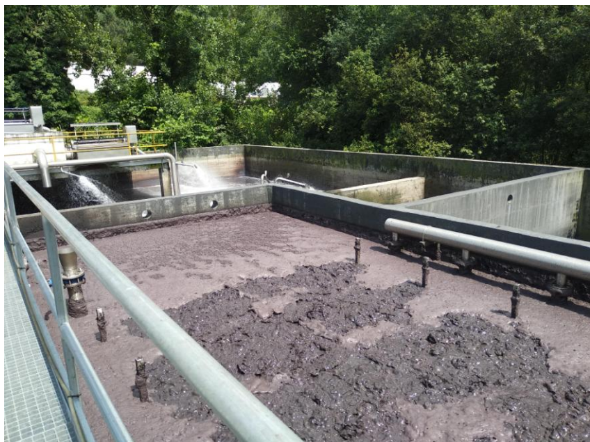
Figure 6.13 MBR system tank, where both biological and filtration processes are done simultaneously.
