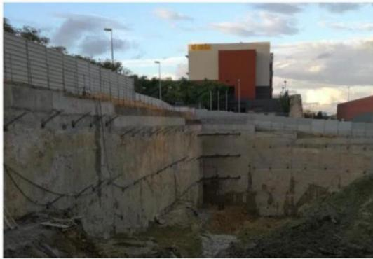
Figure 4 - Props and ground anchors in the diaphragm wall
