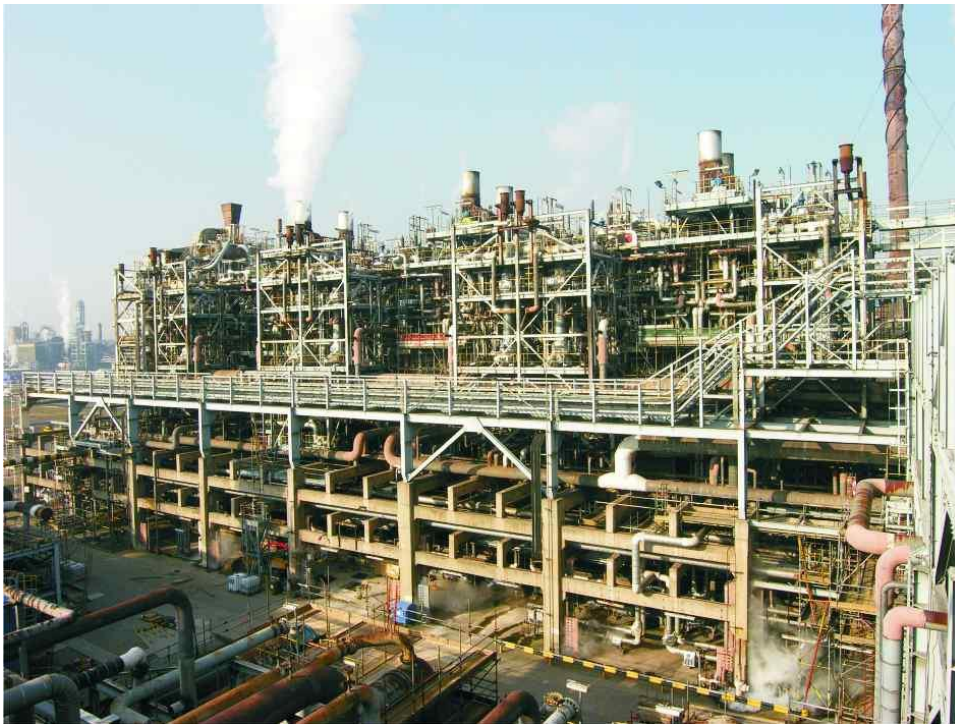
Figure 2.3 - Furnace section of a naphtha cracking plant.
