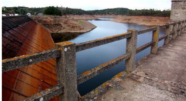
Figure 2.4: Pego do altar Rock-fill dam with a steel layer on the upstream slope. (Source: O Leme - Imagens de Alcácer do Sal).
