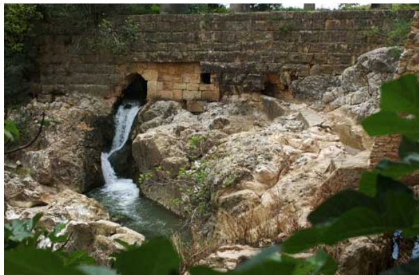
Figure 2.1: Almonacid de la Cuba dam (Parra and Barranco, 2003).
