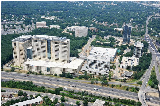
Figure 3-4 – Mark Center building.
