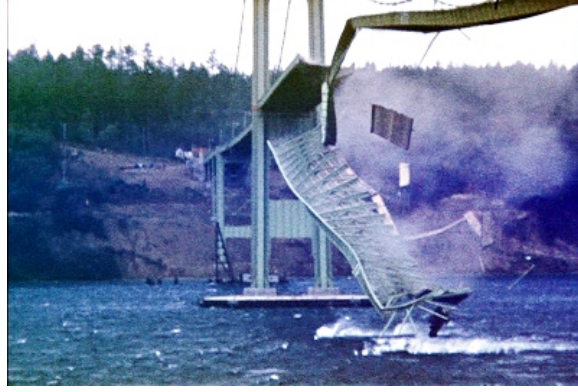
Figure 2.2: Taconama bridge collapse in 1940. Photo taken by Barney Elliot, produced here according to fair use principles; [2]
