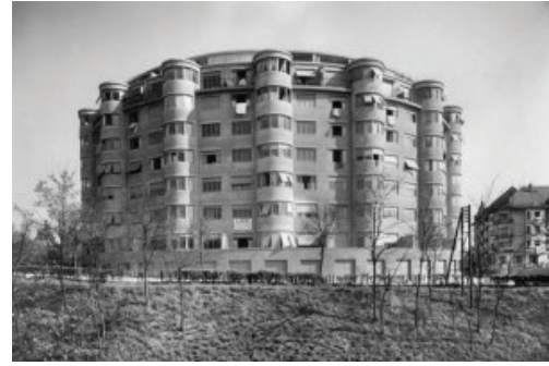
003. Maurice Braillard, Maison Ronde (1927-1930). View of the exterior façade. FBA Archives.
