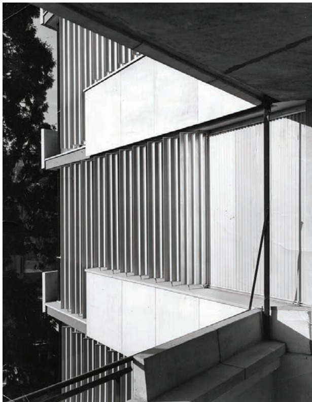
120. View of the façade from the balcony. Photo Klemm.
