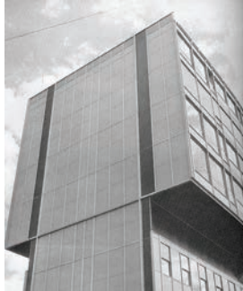
079. Marc J. Saugey, Gare-Centre (1954-1957). View of the curtain wall.
