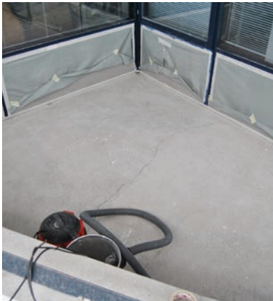
190. 191. Cracks on the ceiling and flooring of a balcony (May 26 th 2014).
