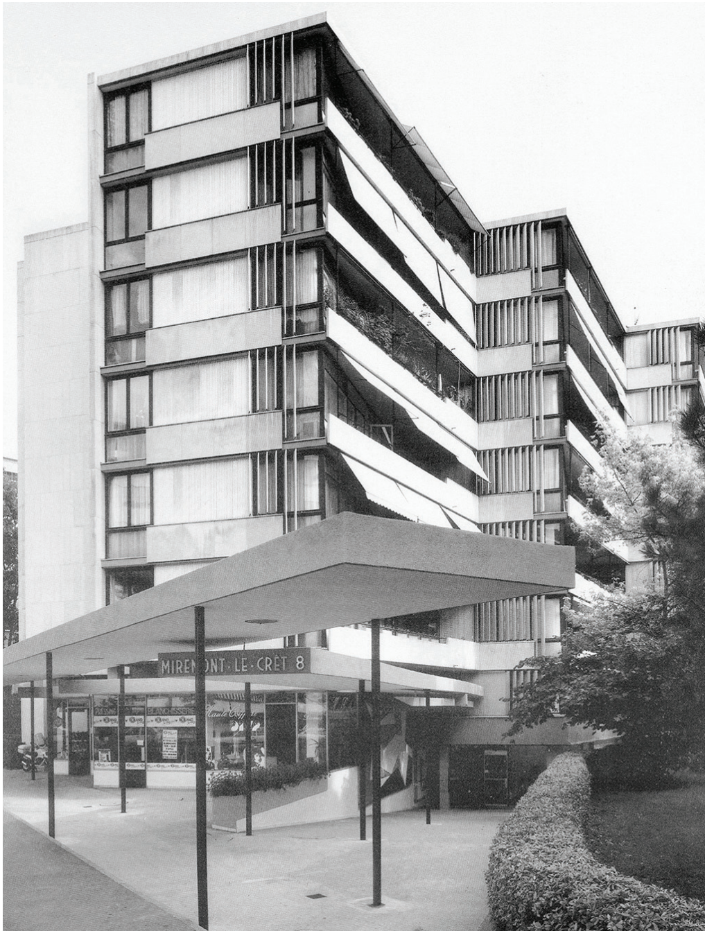
097. Entrance to the building 8 ABC avenue de Miremont. Shops along the sidewalk. Photo Alain Grandchamp.
