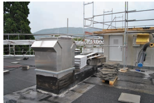
186. New ventilation chimney of the hall (May 26 th 2014).
