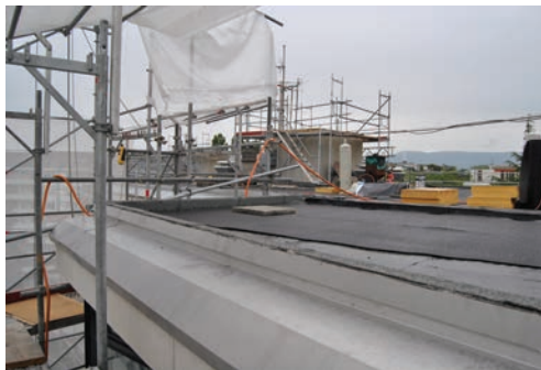
185. Roof being renovated. New profile and flashing cap (May 26 th 2014).
