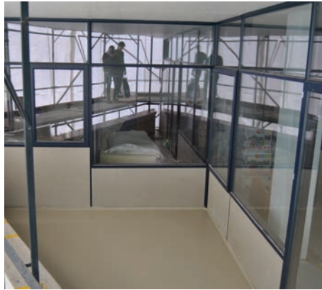
200. A balcony's glazed façade renovated (May 26 th 2014).
