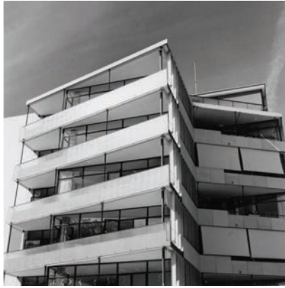
8. South façade. Photo M.-J. Saugey. (Archives IAUG, Fonds Saugey)
