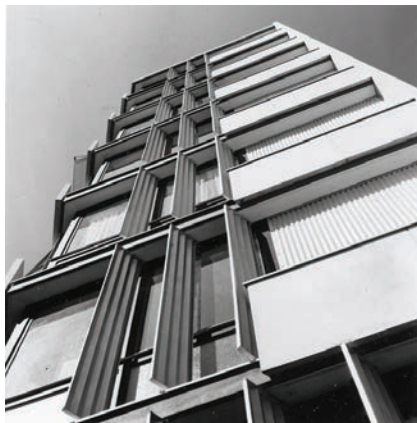
116. View of the façade and its different elements and materials. Photo Saugey.
