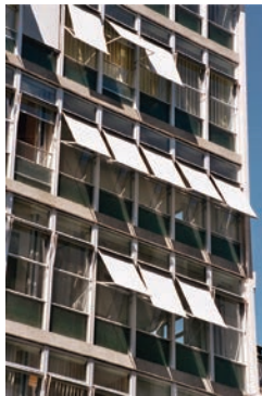
022. Mont-Blanc Centre . Replica panels being installed (2004).
