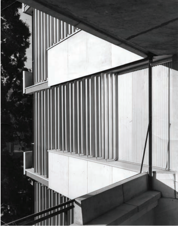
17. Detail of the façade. Photot G. Klemm. (Archives IAUG, Fonds Saugey, no. inv. 3047, cote 205.03.012)
