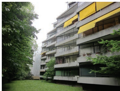
150. 151. Southeast façade (May 26 th 2014). Northwest façade (May 8 th 2014).
