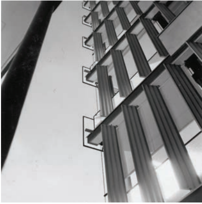
7. Detail of the façade. Photo M.-J. Saugey. (Archives IAUG, Fonds Saugey)
