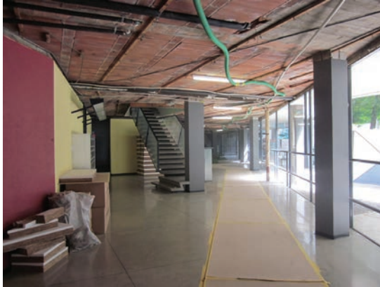
154. False ceiling dismantled. Miremont's hall (May 8 th 2014).
