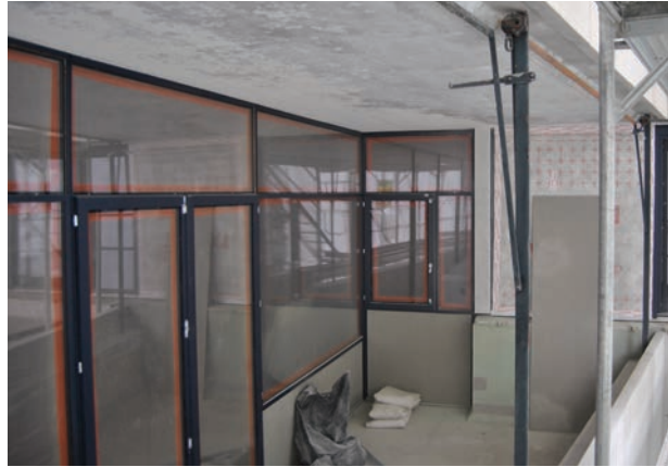
195. Glazing, window frames and opaque panels renovated (May 26 th 2014).
