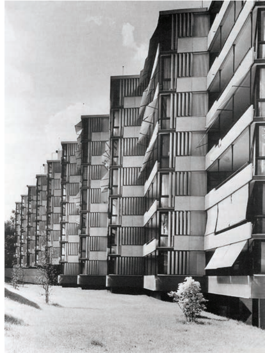
104. View of the Northwest façade.
