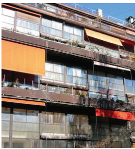
008. Immeuble Clarté . Condition of the building before the rehabilitation (n.d.).
