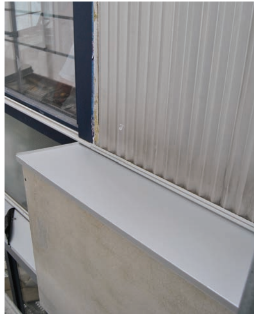
198. Aluminium panel renovated (May 26 th 2014).
