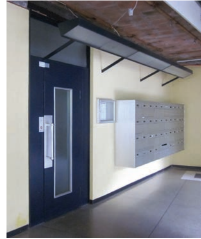
149. Lighting devices on Miremont's hall (May 8 th 2014).
