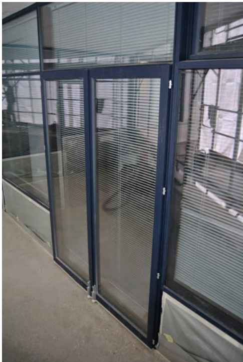
166. Balconies' new casement doors and renovated window frames May 26 th 2014).
