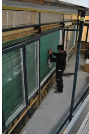
194. Original glazing, window frames and opaque panels removed (May 26 th 2014).
