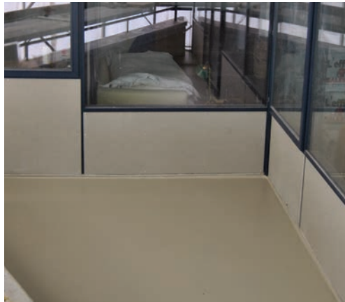
192. 193. Ceiling of a balcony after being treated from carbonation. Flooring of a balcony coated with the insulating resin (May 26 th 2014).
