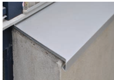
196. 197. New protecting drips in aluminium (May 26 th 2014).
