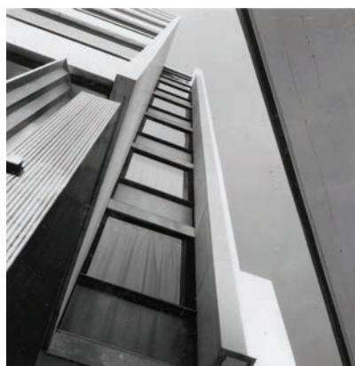
6. North façade. Photo M.-J. Saugey. (Archives IAUG, Fonds Saugey)
