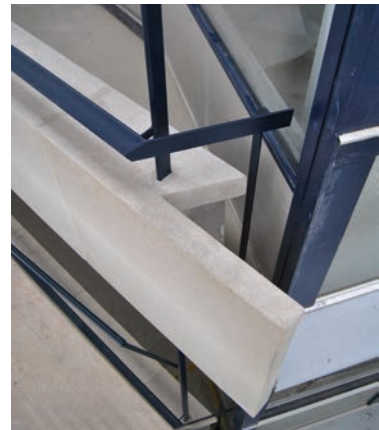
189. Panel restored (May 26 th 2014).
