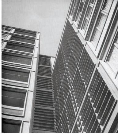
066. Marc J. Saugey, Malagnou-Parc , View of the façade, (1948-1951).
