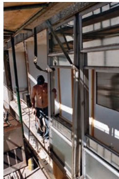
023. Mont-Blanc Centre . Panel being taken down (2004).
