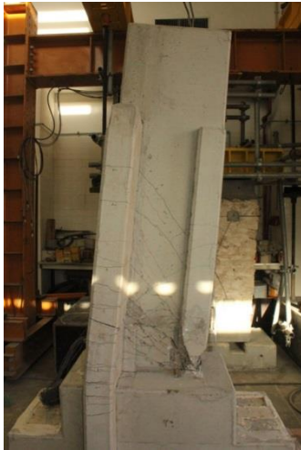
Figure 4.14 – Final deformation of V4 beam
