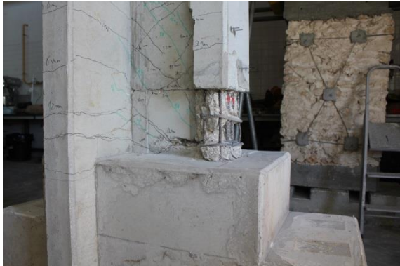
Figure 4.7 – Final aspect of connection (V1)
