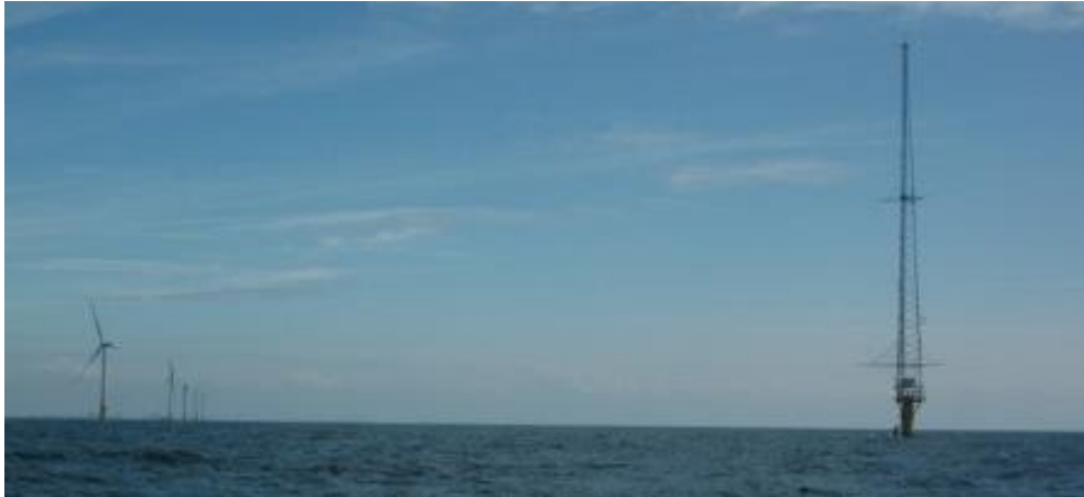
Figure 1: Meteorological mast at the OWEZ wind farm (P.J. Eecen 2008)
