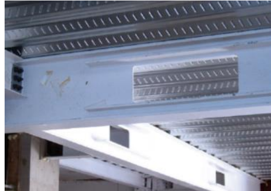
Fig. 2 Rectangular web openings in composite beams.
