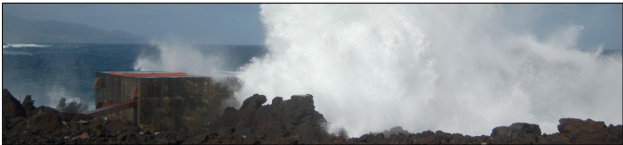
Figure 1 - The Pico Island Power Plant being hit by a massive wave.
