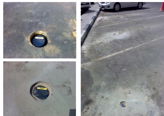
Figure 3.7 - Installation of the wireless sensors.
