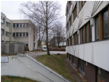
Fig. 47 School buildings to demolish
