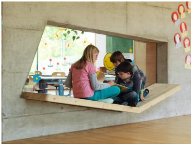
Fig. 24 Niches on the walls between classrooms and recreation area
