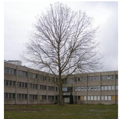
Fig. 51 Building to demolish
