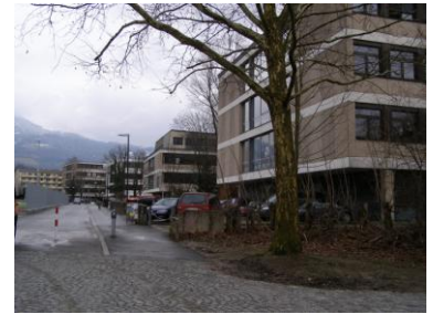
Fig. 50 Secondary school buildings
