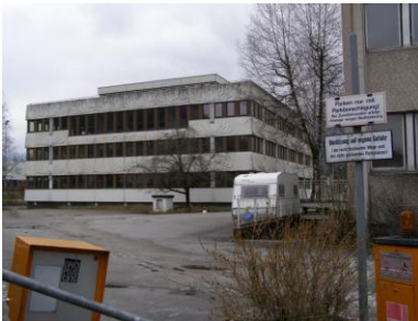
Fig. 59 Building to demolish
