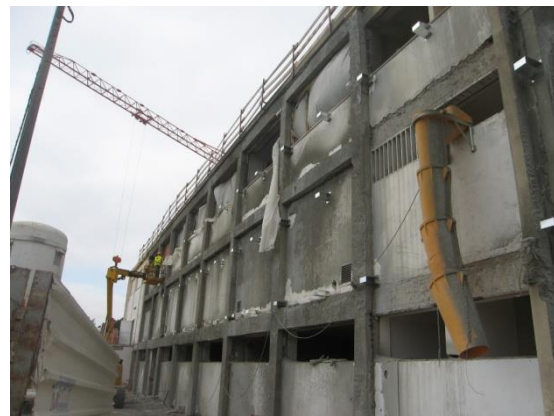
Figure 4 – Gym's seismic strengthening (photo taken in 2010-08-18) – (Laranjeira, 2008-2010)
