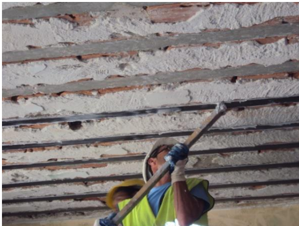
Figure 5 – Applying laminate of CFRP in Santa Isabel School (Jacinto, 2008-2010)
