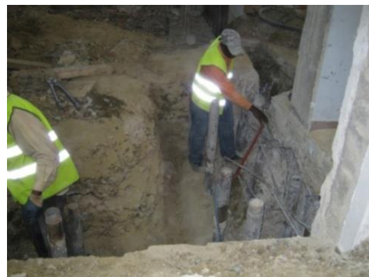
Figure 2 – Reinforced footings with micropiles (photo taken in 2010-10-19 by author)
